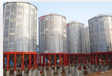
SILOS AT KFL, KERALA
