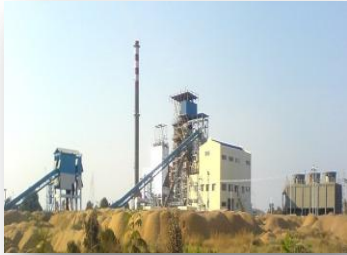
10 MW POWER PLANT FOR VARUN BIO ENERGY
