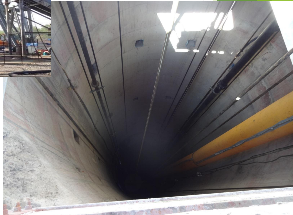
CONCRETE LINED SHAFT - 960 MTR DEPTH 6 M DIA
